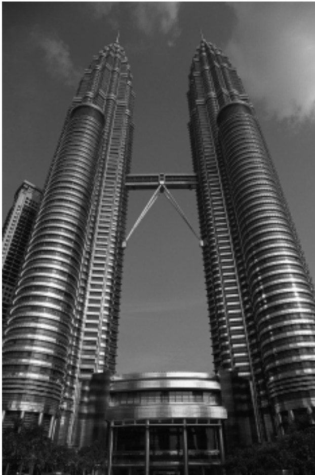
The Petronas Towers, the tallest buildings in the world, are an icon of Kuala Lumpur, which will host the next IGM in May.
